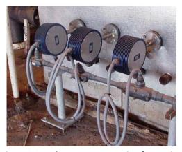
Figure 2-24. Flex sensor connection for service loop, TA version using liquid tight conduit
