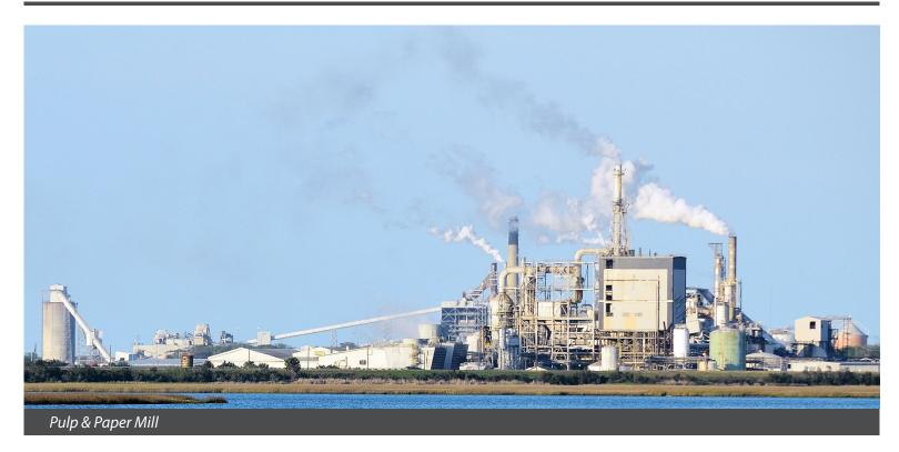
There are more than 20,000 pulp and paper manufacturing facilities worldwide, with an estimated 700 facilities throughout the U.S. and 900 facilities in Europe. Trees used in papermaking are put through a debarker and a chipper, where they are reduced to approximately one-inch wood chips. The wood chips are pressure cooked in a digester and become pulp, which is refined, turned into slush, and screened. Screening drains away liquid, and the resulting pulp is pressed into paper.
