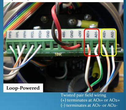
NOTE: The 4-20 mA connections are polarity sensitive, if the wiring is reversed the output will be zero
