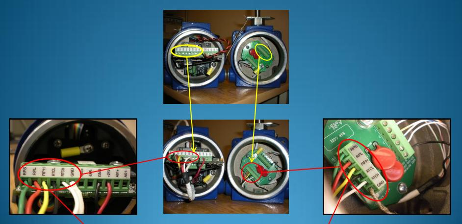
The sensor wires should terminate at the electronics enclosure and the sensor enclosure at the terminals marked RPS / RPL / RPH / RTCL / RTCH as shown and the braided shield should terminate at the GND terminals
