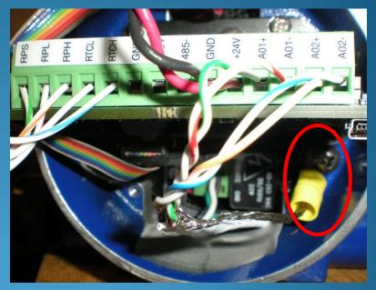
Typical 4-20mA field wiring termination
