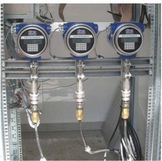
Cable Gland Example with Braded Shielded cable on a TS configuration.
